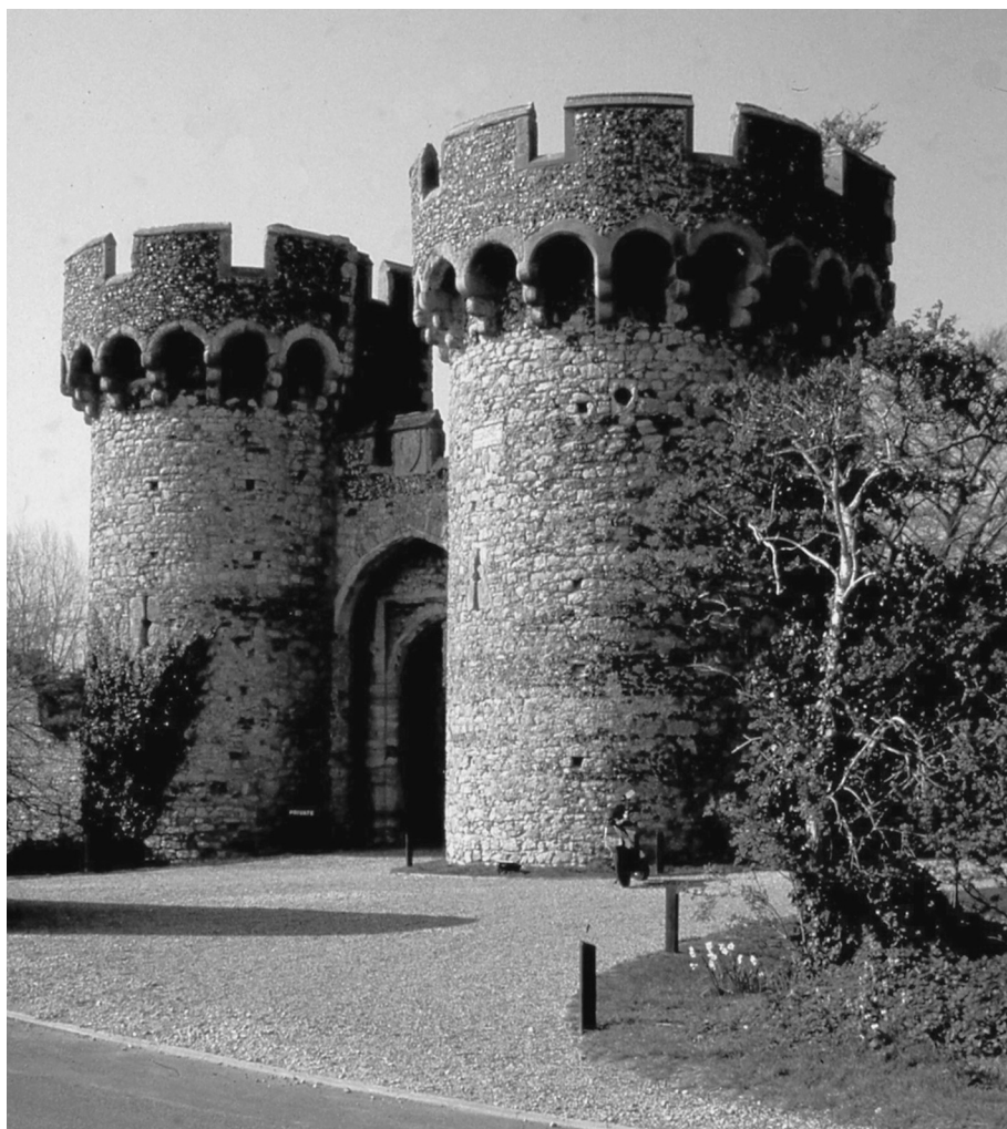
Cooling: Outer gatehouse from the SE. 1381.
